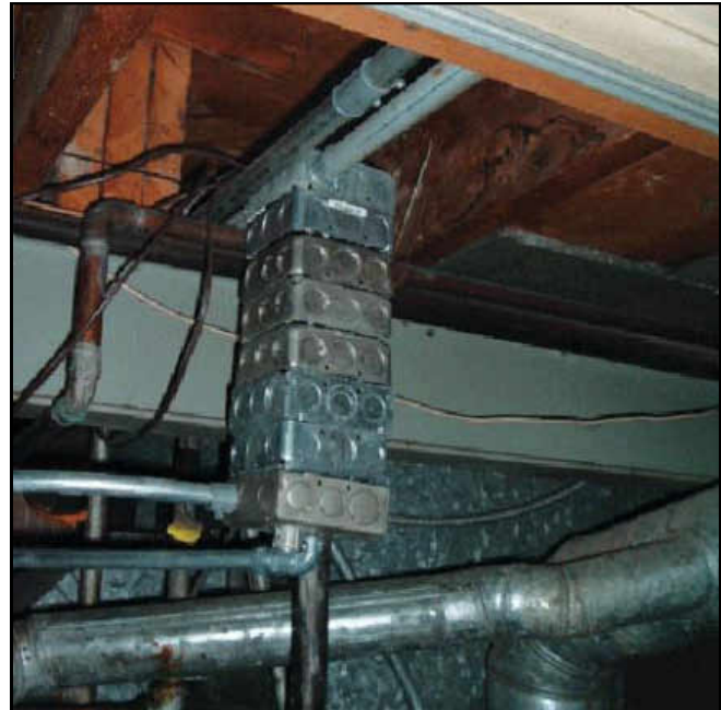
Missed it by a foot, why not use a bunch of spare electrical boxes?
