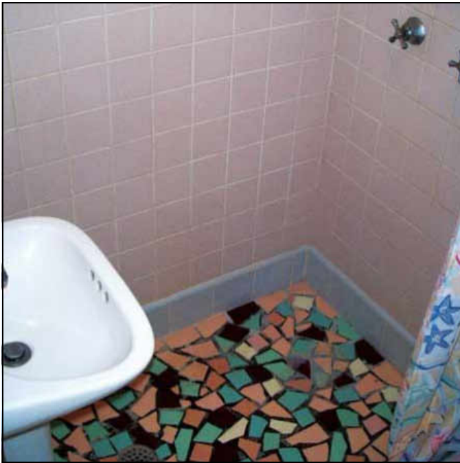
No place to put the sink? Then let's make it a combination sink and shower
